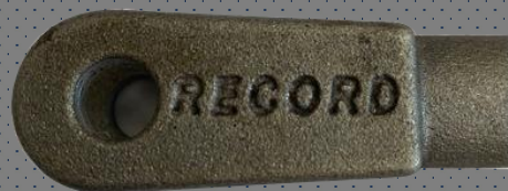
Investment Casting Clevis in Pendulum Clasp made by Weser
